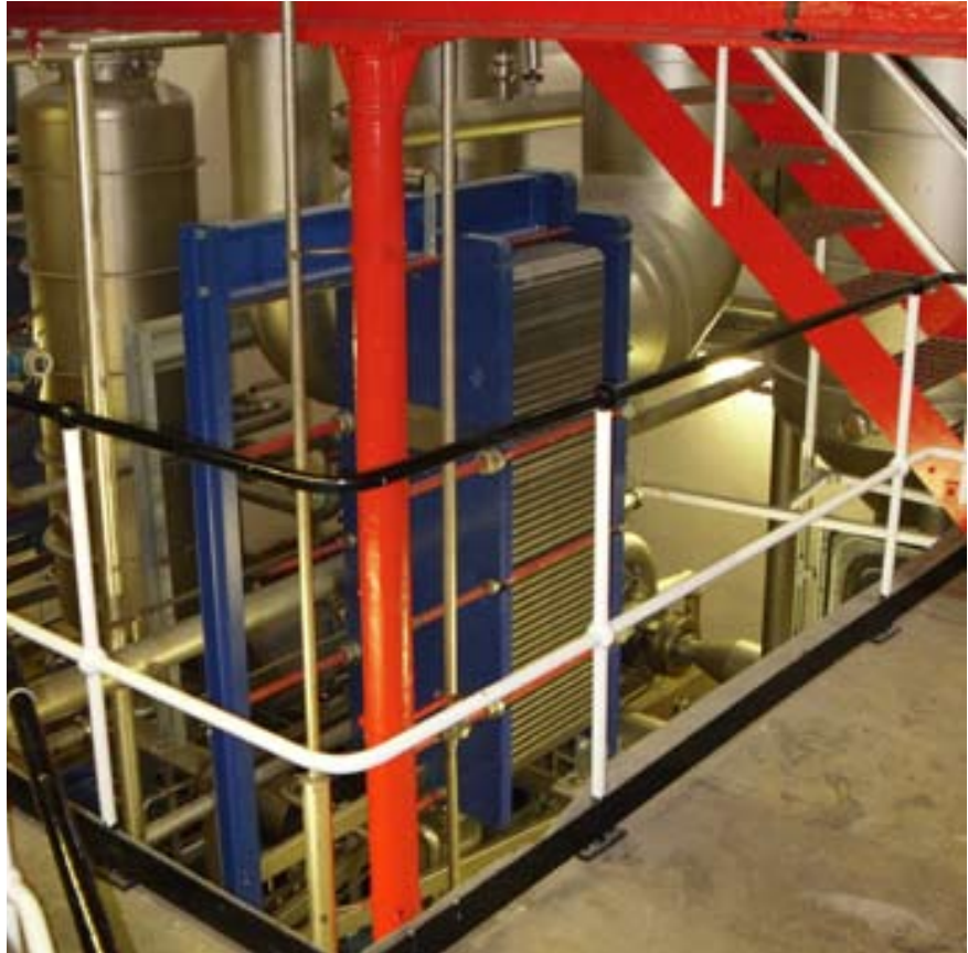
An Alfa Laval plate heat exchanger in the evaporation system. Glenfarclas invests in the latest technology to maintain the quality of its products.
